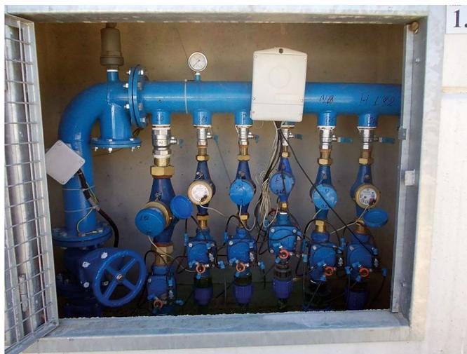
Drip irrigation was likened to a "silver bullet" by some international publications, seen as having the ability to free up water resources and rebalance depleted basins through water savings. Above, a metering cabin in the Acequia Real del Júcar. / Mar Ortega
