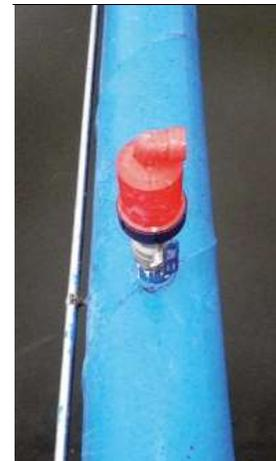
*Detail of a valve in the pressurised irrigation system in the Acequia Real del Júcar. / Mar Ortega*
