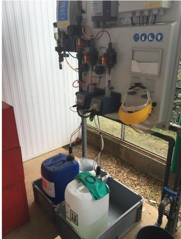
Figure 1. Sodium hypochlorite injection system using an electric pump and reservoir water at a UK ornamental grower's nursery.
